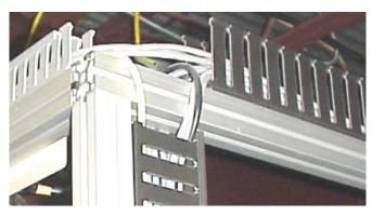
Figure 49: Wiring Channels
