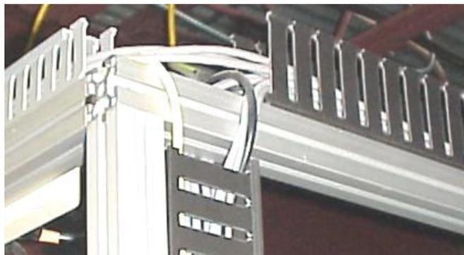
Figure 49: Wiring Channels
